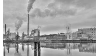
Figure 4.27: Factories besides a body of water. Many organisations aim to use drones to scan air pollution in the surrounding areas.
