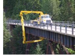
Figure 4.5: Bridge inspections with a snoopers truck [401] (2016).
